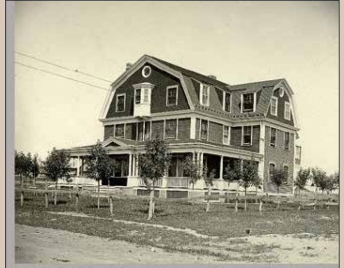
The Smith Hospital. This view from the southwest (corner of Clough and Billings Streets) shows the gambrel roof lines. Not visible in any known images is the glass roof over the operating suite which located on the northern side of the building. Note the profusion of trees - Drs. Smith planted nearly their lots, 2 of which appear to survive to present day. Dickinson Museum Center, Osborn Photo Collection.
