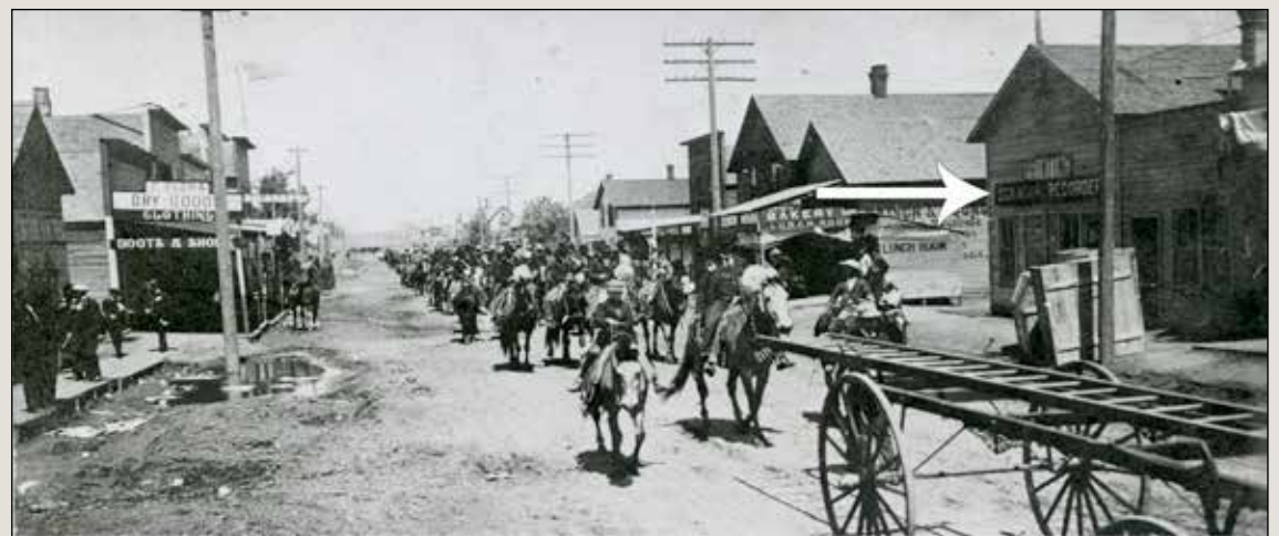
The Dickinson Recorder office when it was on the east side of Sims Street in the late 1890s. A parade is going down the street. Image from SWNDDA #2010-018-203.
