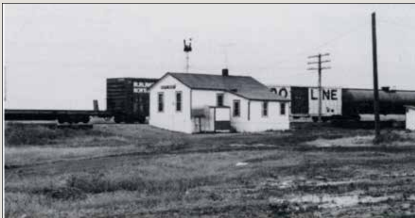
South Heart Depot sometime after 1970. Note the addition which housed the washer, galvanized bathing tub, water heater and chemical toilet. The outhouse which served the Depot prior to the addition can be seen to the right. The function of the smaller lean-to addition is unknown.
