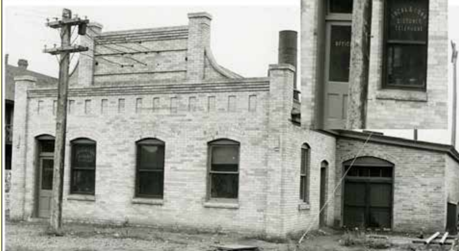
The original power house /telephone exchange building on the south side of West Villard Street. Note the 'Local & Long Distance Telephone' door signage and the plants in the adjoining window – perhaps placed there by the exchange's female operators.
