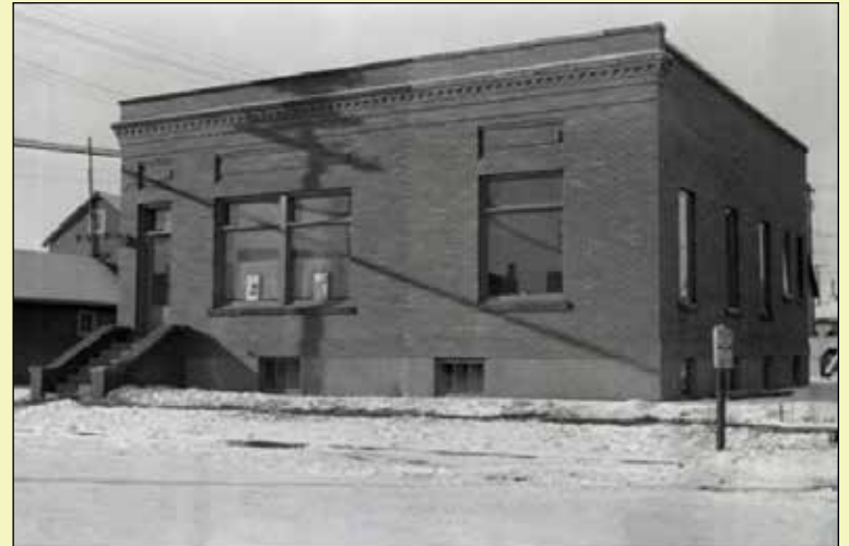
The North Dakota Independent Telephone Co.'s exchange building on 3 rd Ave. W. The left half of the building is original to 1910 (note slight difference in brick color). This was later part of the Northwestern Bell Telephone System. Photo dated 1949, Dickinson Museum Center, Osborn Photo Collection.
